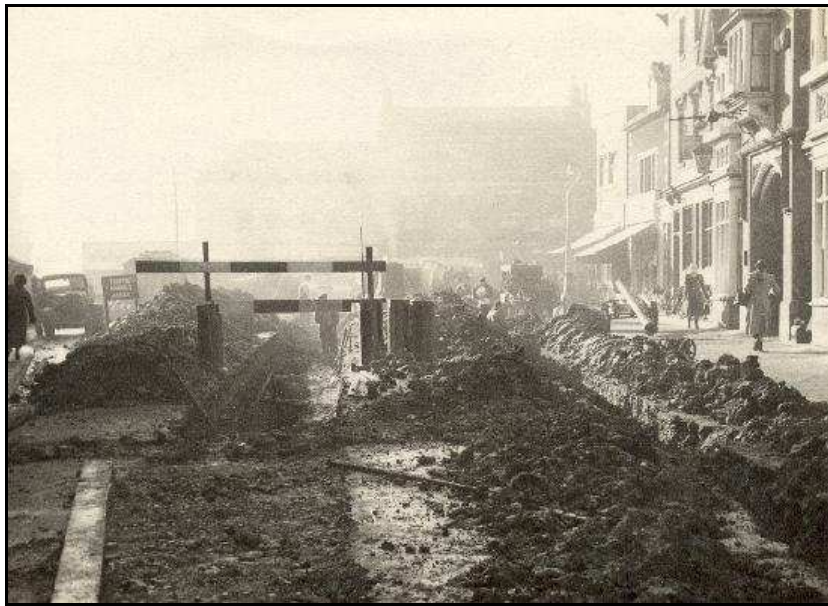
A new sewage system being installed in 1960
