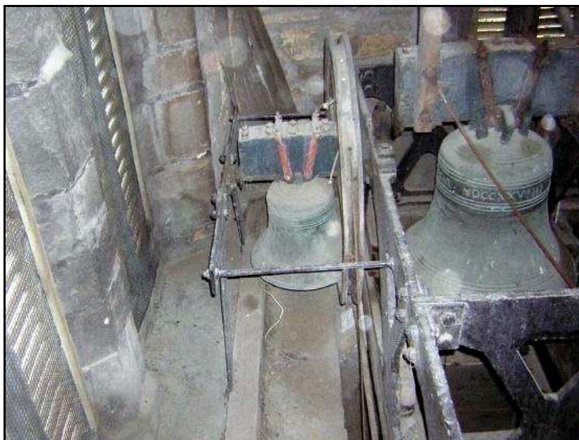
Inside the bell chamber – photo courtesy Jim Jones
